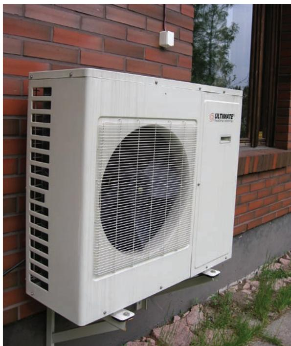
*An outside unit of an air-source heat pump.*
